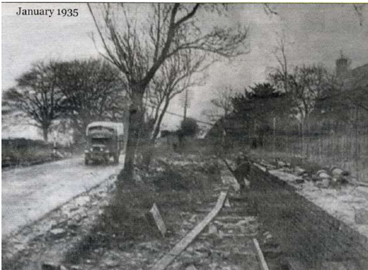
Swindon Advertiser : 'RICHARD JEFFERIES' WALL—A photograph of the work in progress on the setting back of the wall of the Richard Jefferies' house at Coate, Swindon. The beginning of the new wall is seen on the right, its original position is marked by the line of trees, which were inside the fence, its removal is due to a road widening scheme at this point, sentiment having had to give way to safety.'
